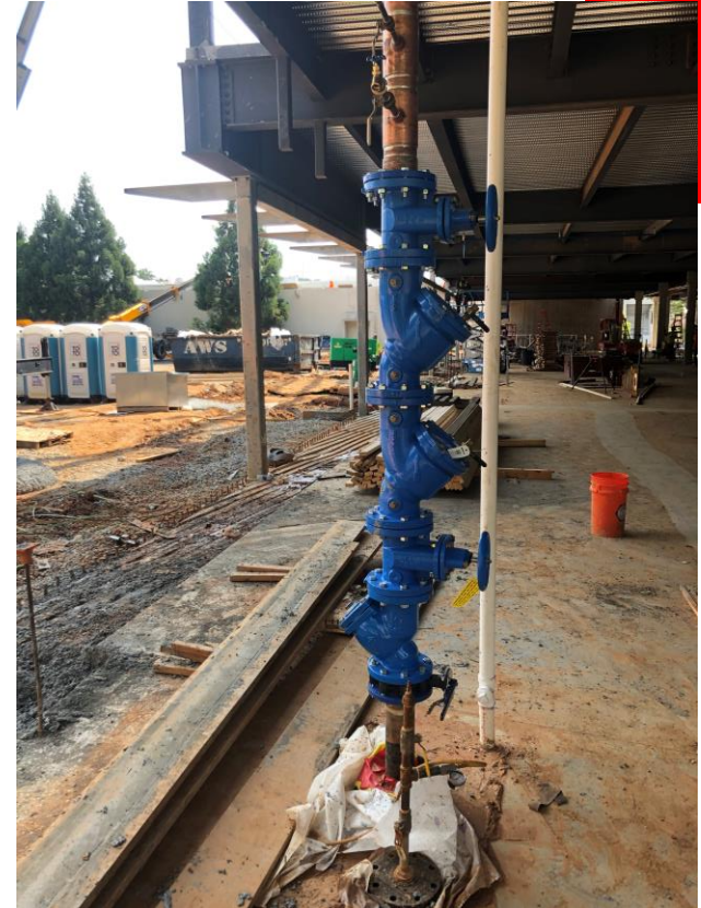
Water Riser Valves Installed
