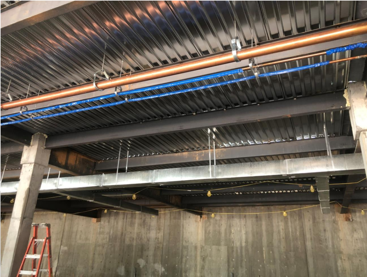
MEP Overhead progress at New Additon
